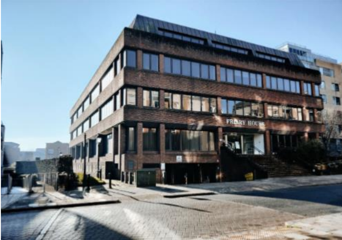
Figure 6 – Existing Building from Briton Street Compared with New Building from Briton Street
